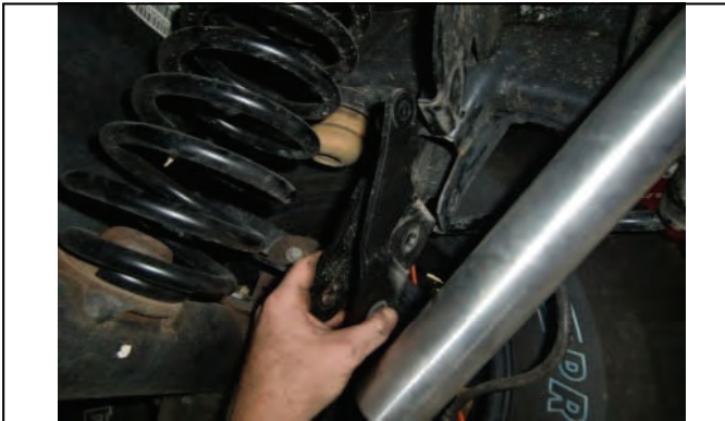
Remove track bar and ReadyLIFT rear drop bracket
