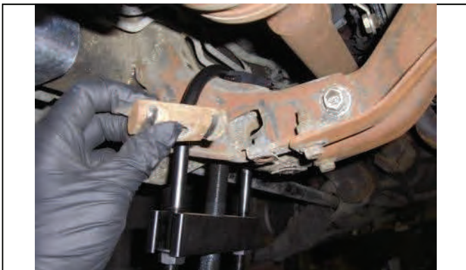
Adjust tool enough to remove keeper block
