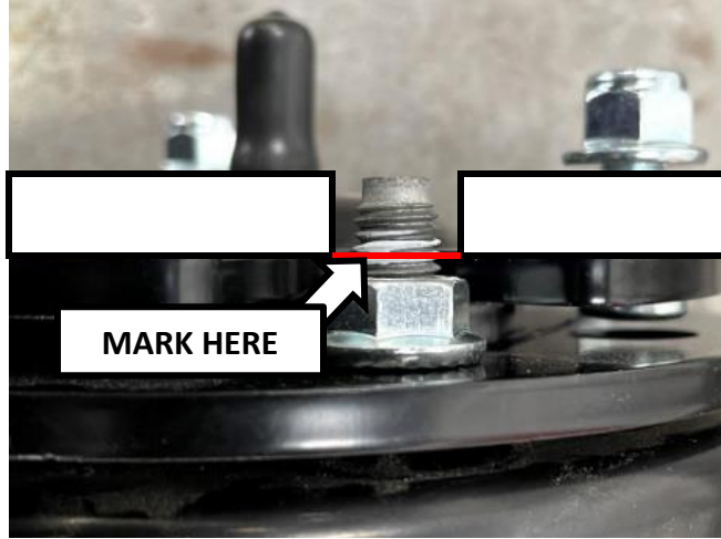
Figure 17: Marking the Strut Top Studs
