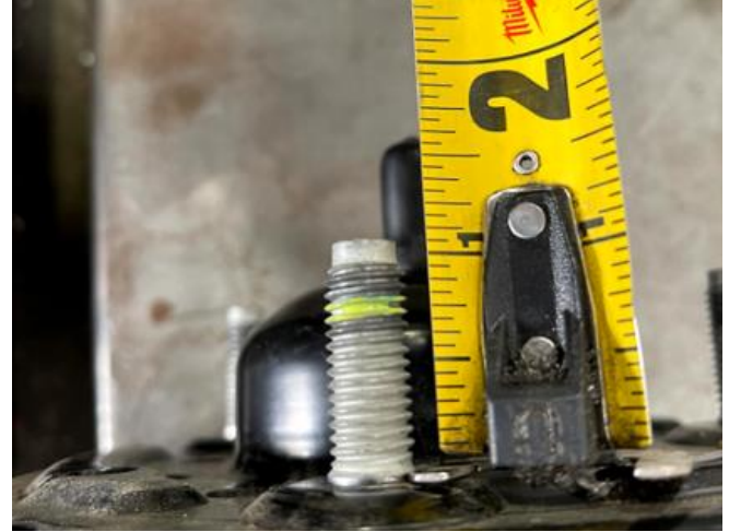
Figure 18: Measuring the Strut Top Studs
